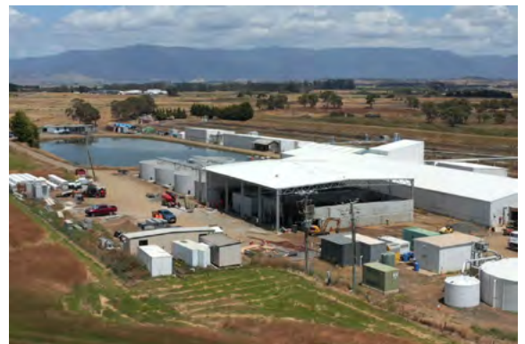
CRESSY III DURING THE CONSTRUCTION PHASE.
