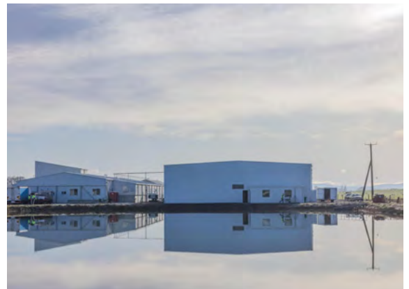
CRESSY III CONSTRUCTION COMPLETED AND ALL SHIP SHAPE.
